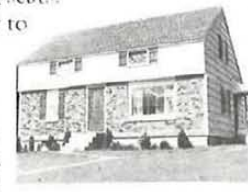
12 Private Road Lane
